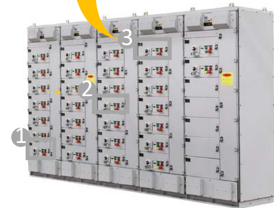
Obstructed Access/Poor Visibility
