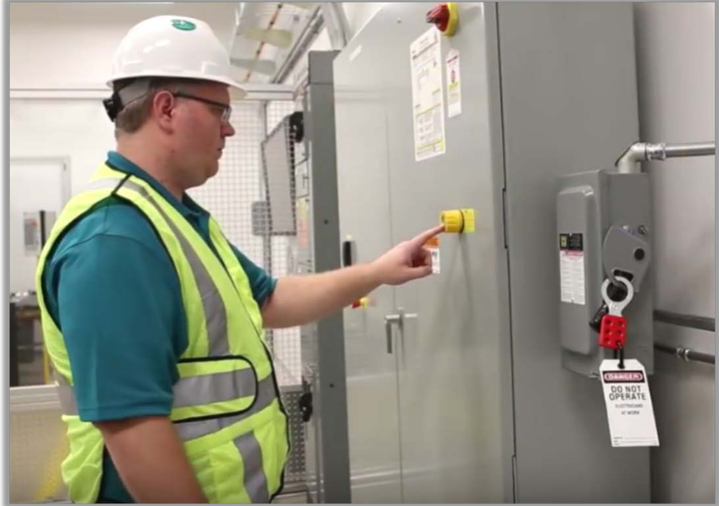
Using a Permanently-Mounted Absence of Voltage Tester (AVT)
