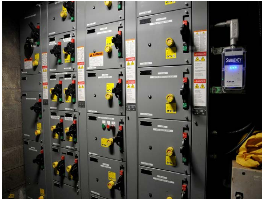
MOTOR CONTROL CENTER (MCC)
